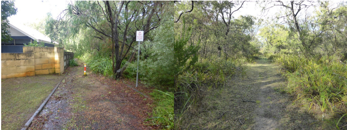
Figure 3-4 Emergency access off Lagoona Place that could be improved with new hot mix.
