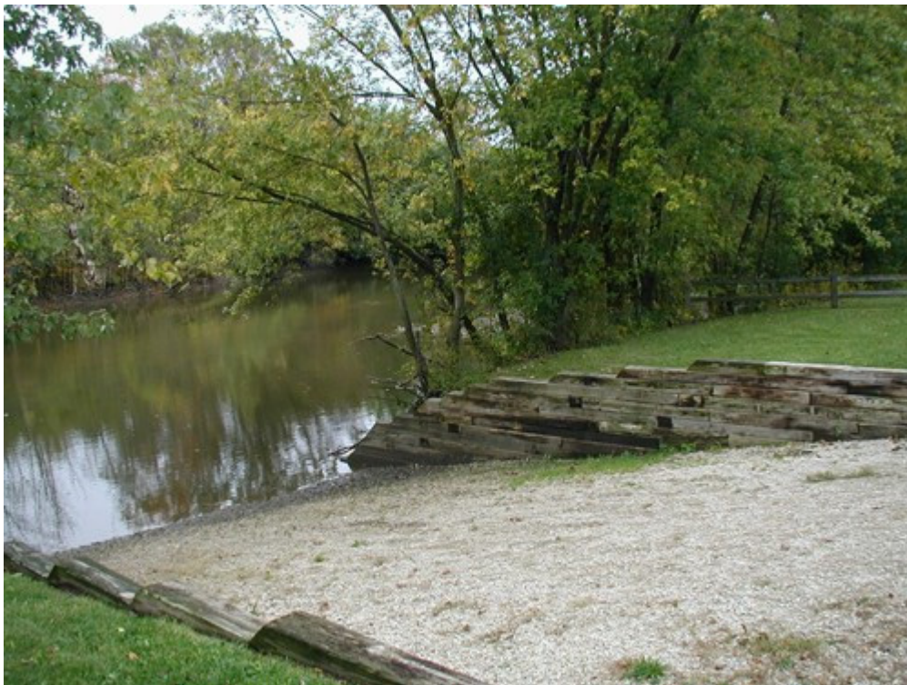
Figure 3-20 Example of graded access to the water mark. Note that retaining walls would still be required at the bank cutting. Source: https://www.lcfd.org/launches/
