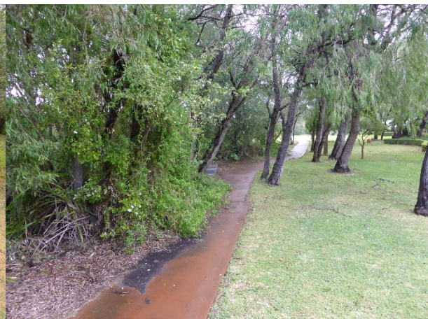
Figure 3-3 Existing path near Stone Street requiring maintenance.
