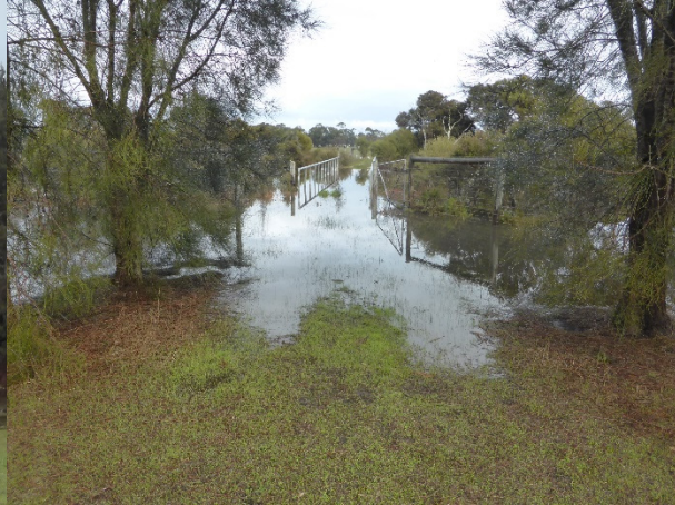
Figure 3-14 Foot bridge (WP 2)
