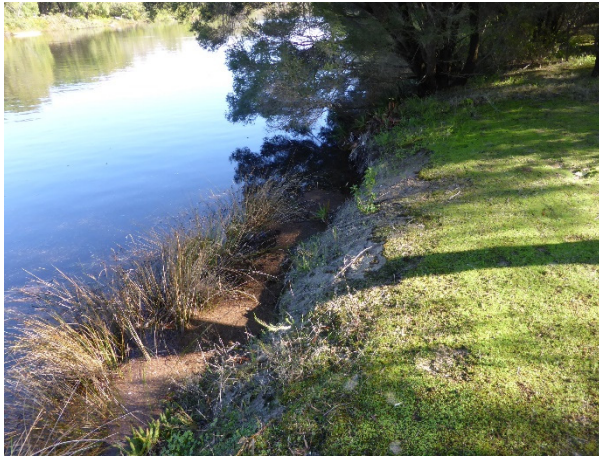
Figure 3-8 Example of erosion at Mc Quade Park (Campion Way) due to loss of stabilising foreshore vegetation.
