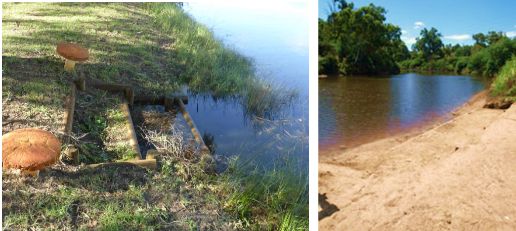
Figure 3-19 Examples of stepped retaining walls that could be enlarged for canoe access, or as a fishing platforms in degraded areas.
