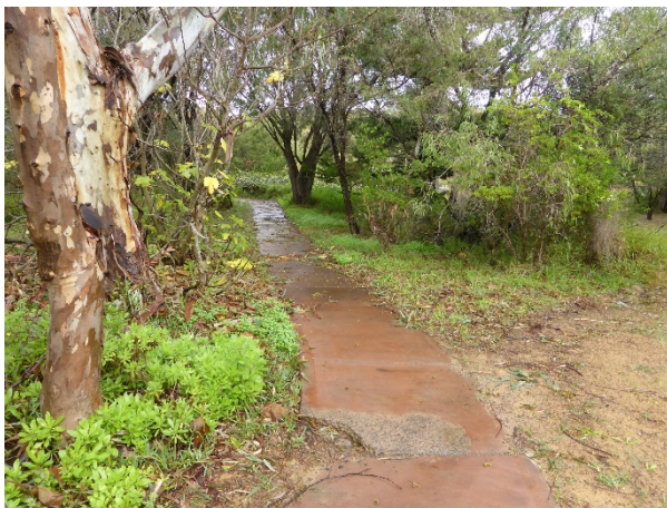
Figure 3-2 Existing path south of Geographe Close needing repair.
